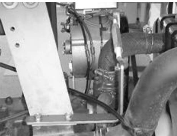
Bracket used to support to Power Generator and to provide a mechanism for V-belt tensioning
